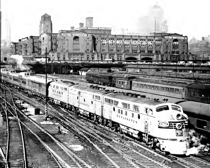
The multiple railroad lines converging upon Chicago make it possible for the city's industries and businesses to ship their products to every corner of the land.
